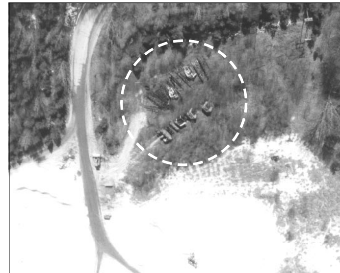
Abandoned mining equipment in November 1997 located in Cell 1.
