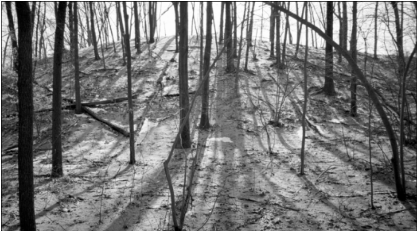
Sand blown from the active face of the mine has covered the north slopes of the dunes north mine and adjacent to Rogers Creek. The deposits are already two inches deep threatening vegetation on the slope. Sand has reached the creek threatening this natural trout stream.
